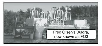
Technology: No tidal technology. FO3, the Fred. Olsen Group's wave energy device, exists only in scale model prototypes, though the FO3 is one of three technologies selected for Wave Hub. It looks like so many giant eggs bobbing under an offshore oil platform. The vertical motion of the eggs is converted to rotary motion which turns a generator.
